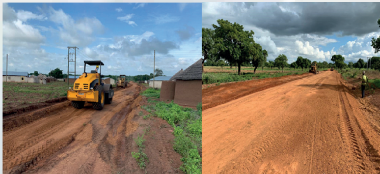
Access Road to the Site Repaired
