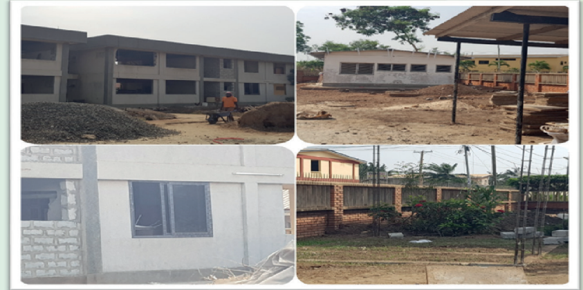
Renovation Work - Tema
