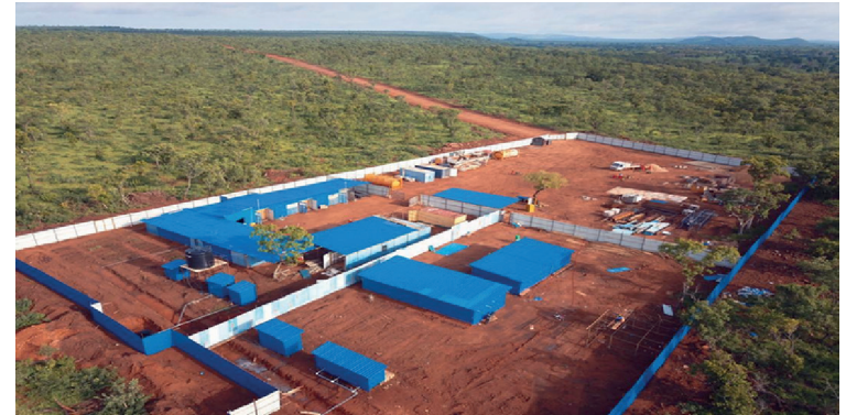
Temporary Workers' Camp Completed
